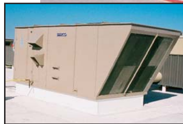
A natural gas-fired SEMCO Revolution™ desiccant dehumidification system was retrofitted into this Georgia elementary school.
