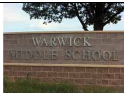
The new Warwick Middle School sits on 172,000 square feet in Lititz, Pennsylvania.
