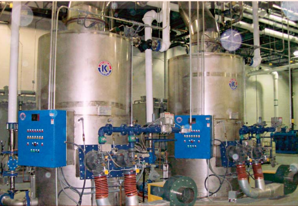
Multiple units can be combined to increase capacity or to provide diverse hot water temperatures. Photo courtesy Kemco Systems.
