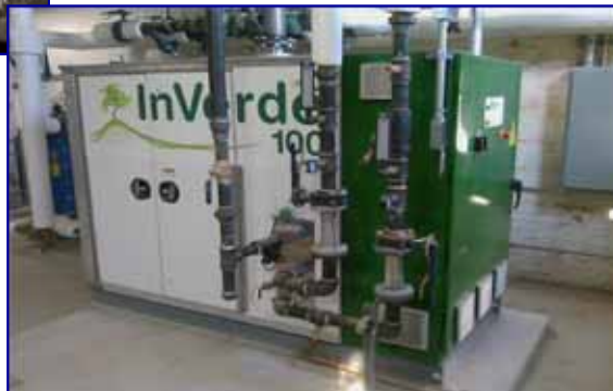
The CHP demonstration at Frito-Lay North America, Inc. in Yankee Gas service territory provides 99% of the plant's power, and operates at a CHP efficiency of 70%.
