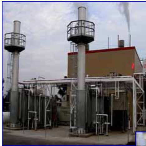
The CHP demonstration at Frito-Lay North America, Inc. in Yankee Gas service territory provides 99% of the plant's power, and operates at a CHP efficiency of 70%.
